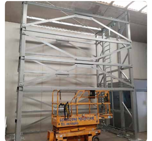
REINFORCED EARTHQUAKE-RESISTANT STRUCTURE
