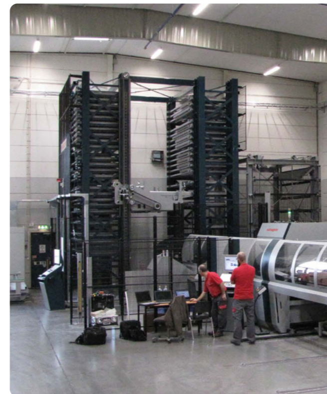
Automated storage system for metal sheets stacked on trays (mechanical sector)
