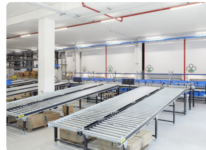
CONVEYOR BELTS AND ROLLER UNITS
