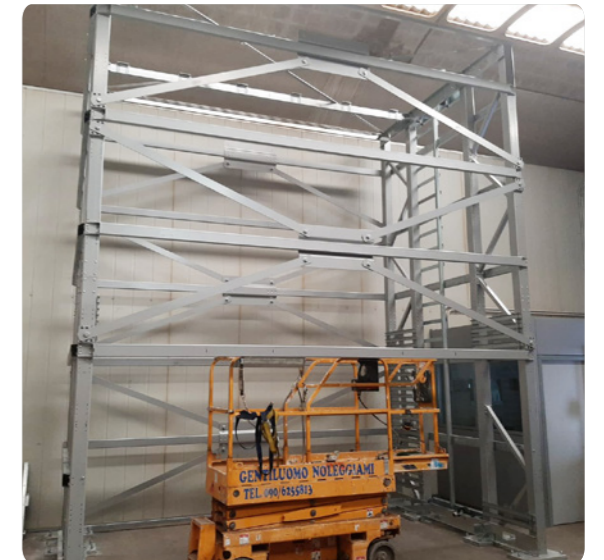
REINFORCED EARTHQUAKE-RESISTANT STRUCTURE
